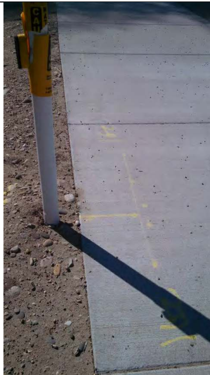
Photograph 29: Natural gas pipeline marker observed along N. Whitewater Park Blvd. Markings indicate the pipeline runs parallel to N. Whitewater Park Blvd. and does not traverse the site.
